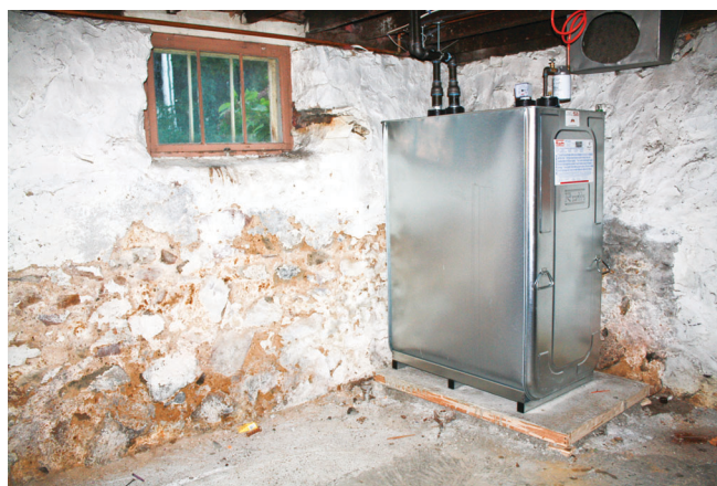
The new Roth double-shell tank looks more like an appliance than a tank.
