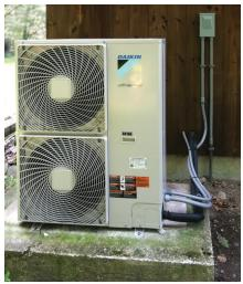
It can also provide domestic hot water (DHW) through an indirect water heater. Because it is a heat pump, the whole cycle can be reversed to provide chilled water (41°F-70°F) for cooling. They have been in Europe for the last five to ten years and continue to grow in popularity.
